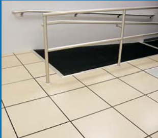
Raised Floor Environment
